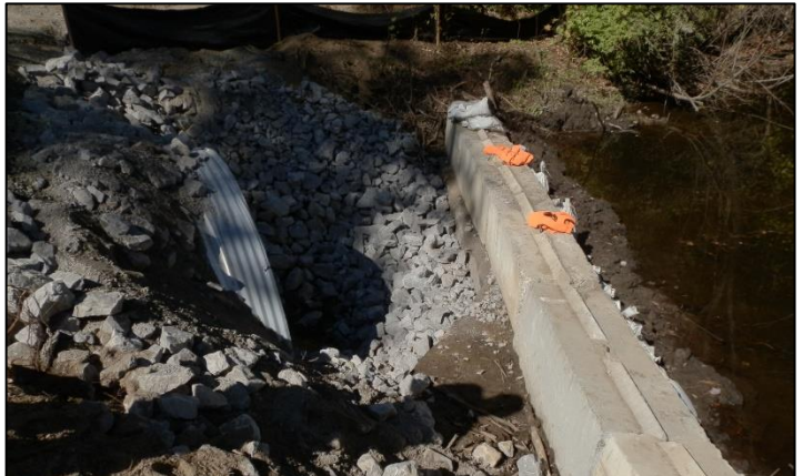
During installation a coffer dam was constructed to divert flowing water around the work area.
