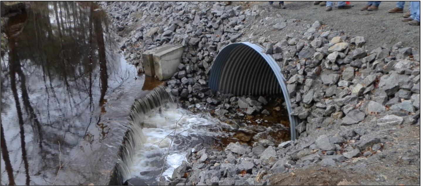
A 7 foot squash culvert pipe was installed. This size pipe can easily handle the stream flows for up to a 100 year storm event. Rock head and wing walls will create a surface that will resist erosion and keep water in the existing channel.
