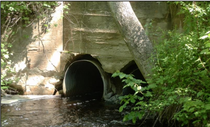
Water was flowing around and in-between previously installed culverts.
